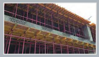
Air cargo terminal at "Domodedovo" airport, floor slabs up to 22 m and load up to 6 tons to 1 m².
